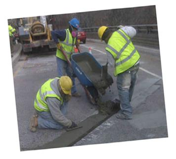
**Fastcrete** is a proportioned blend of dry aggregate, graded sands, cement and set accelerating additives to give a concrete mix suitable for all general concreting applications where fast setting characteristics are required.
